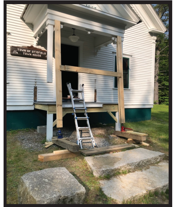
The front entrance of the Town House as repairs begin
